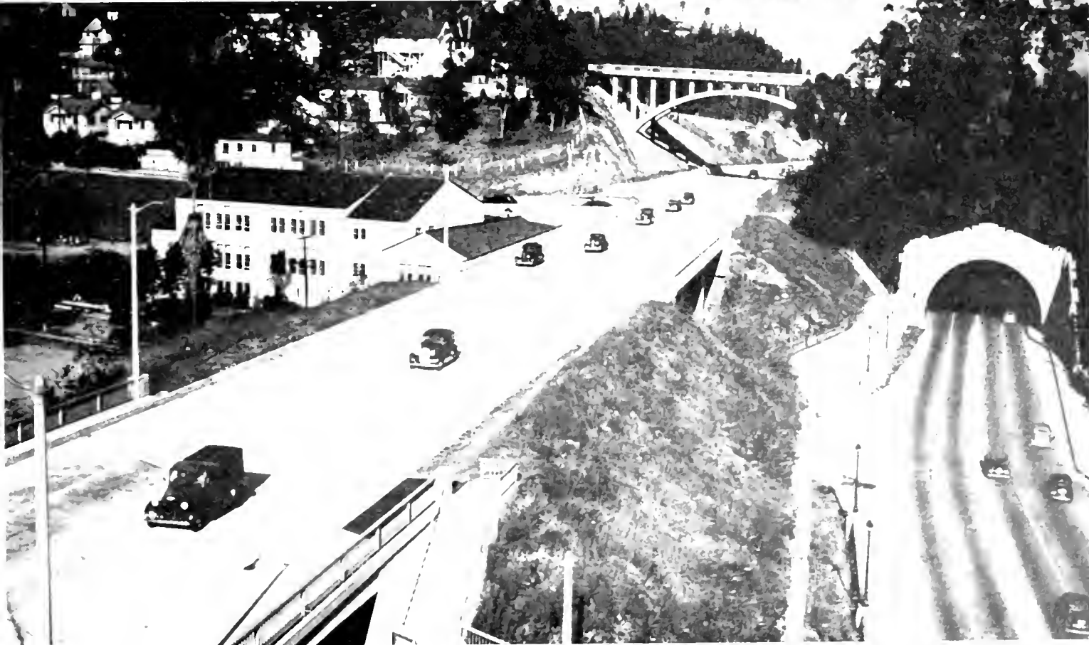
At top southbound traffic is approaching Los Angeles on new Arroyo Seco Extension and third level on the E. 10th Park City Highway. In background, Old road at left. Below—Southbound traffic passing under Park Row Bridge and Northbound traffic entering tunnel.
